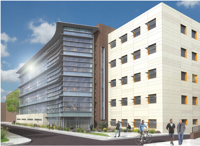
New NJCU Science Building (Located Next to Michael B. Gilligan Student Union)
